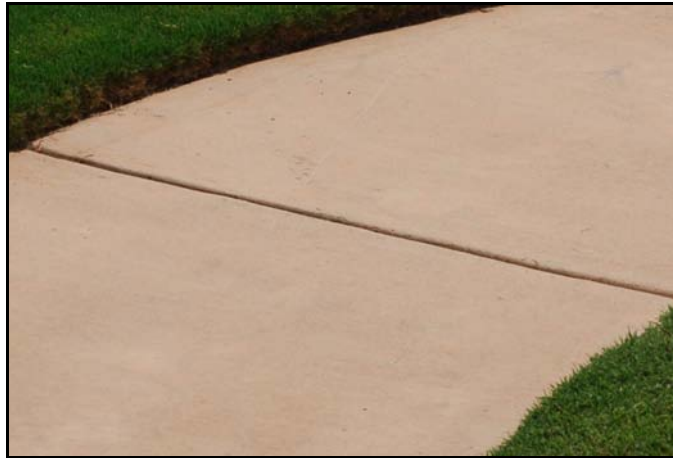
Expansion Joint in Concrete Walkway
