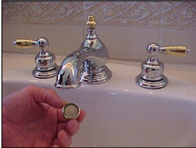
Remove the Aerator Screen to Repair Blockages
