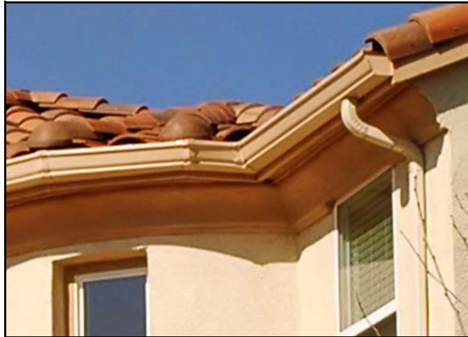
Gutter and Downspout
