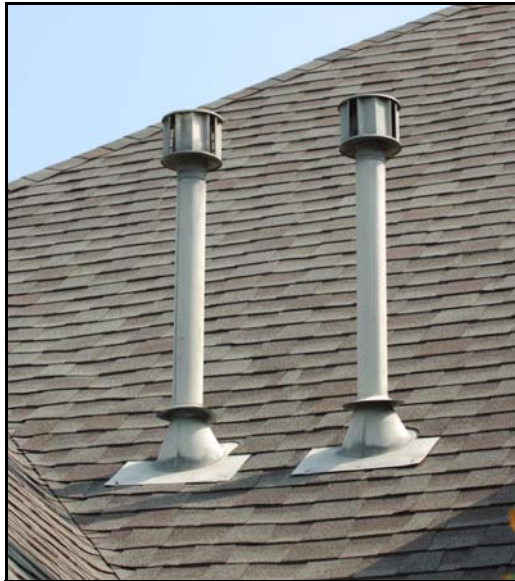
Example of roof penetration flashing
